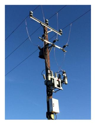
Three pole-mounted HV capacitors are installed as part of Smart Street, two in the Egremont trial area and one in the Wigan trial area. The pole-mounted HV capacitor banks are supplied by ABB and are:
