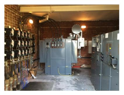
As part of Smart Street, Electricity North West has installed five distribution transformers with an on-load tap changer (Figure 11). These transformers are a standard distribution transformer with the addition of:
