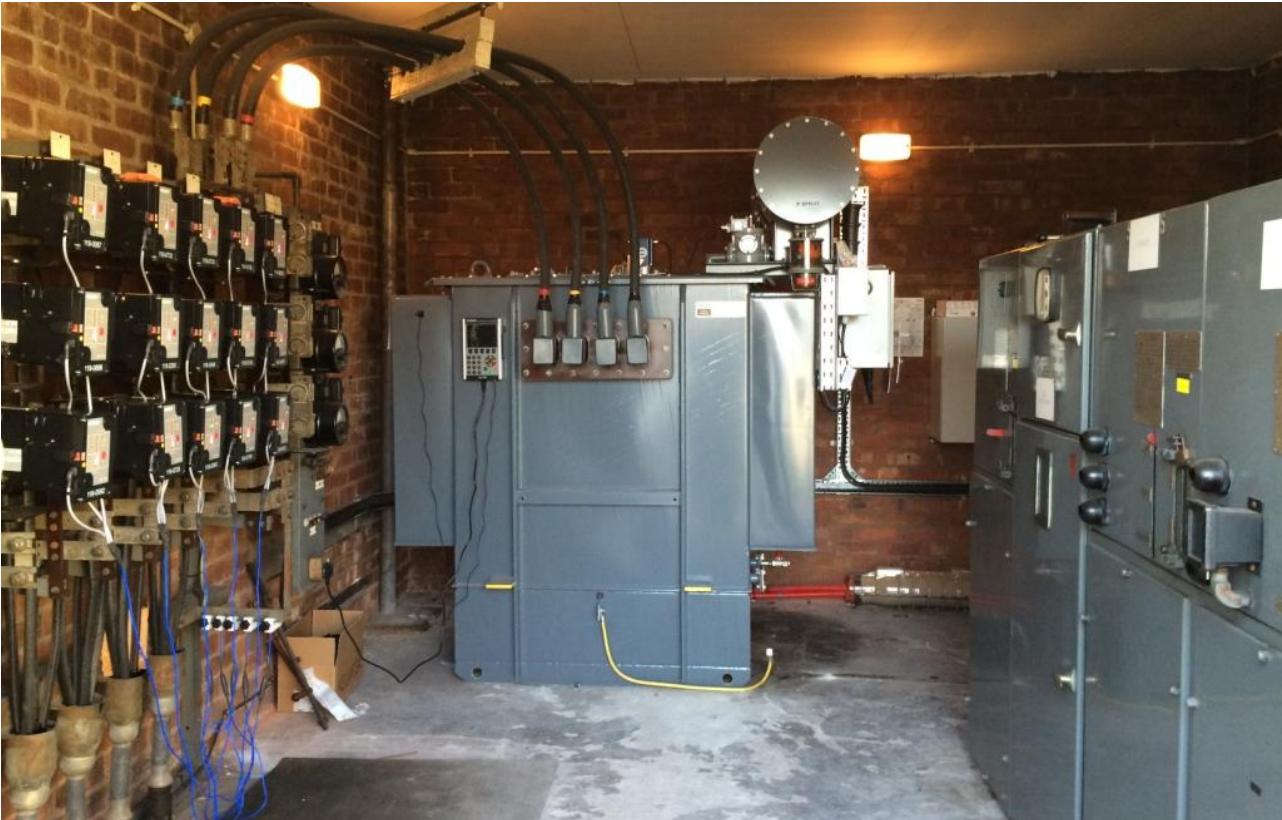
Figure 6: Vauxhall Rd OLTC transformer installation
