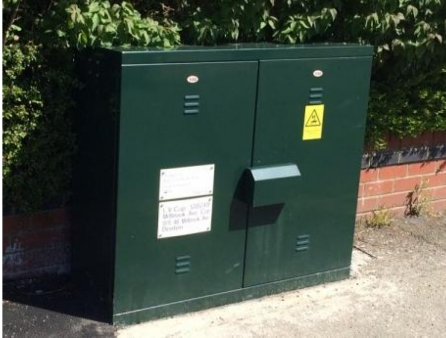
Figure 4: LV capacitor installation, Denton East.
