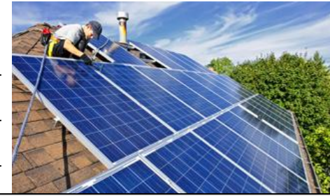
Photovoltaic Panels (PV)
