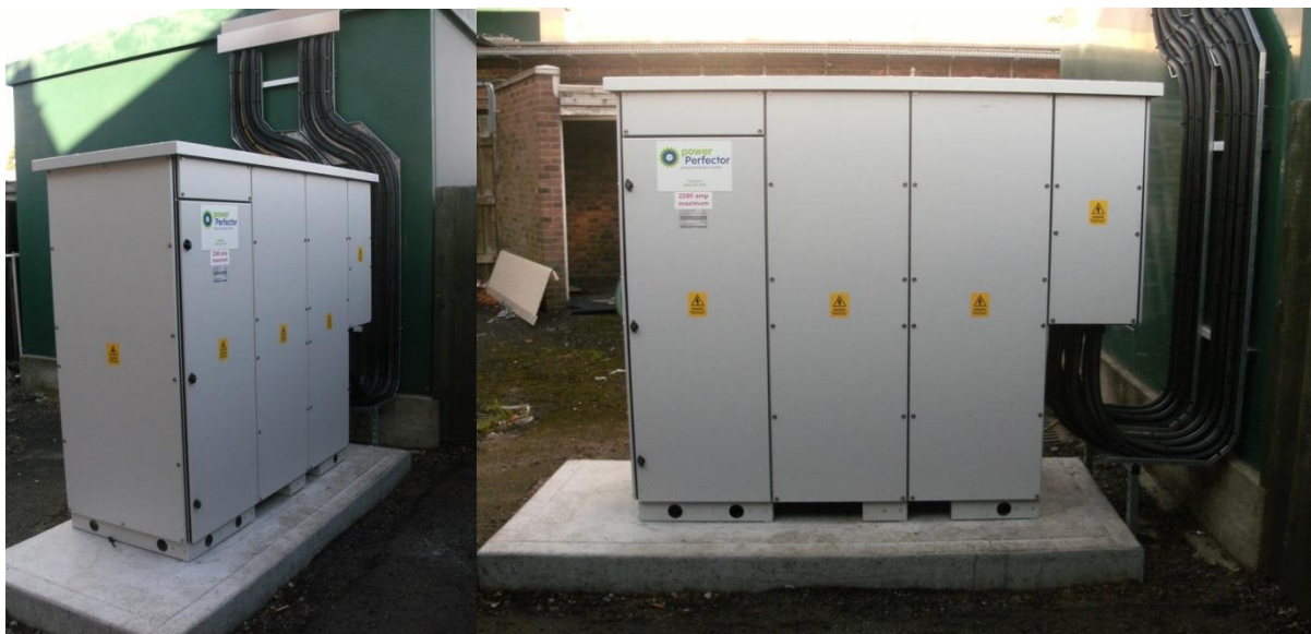
Figure 55: powerPerfector unit installed at Edge Green Lane substation
