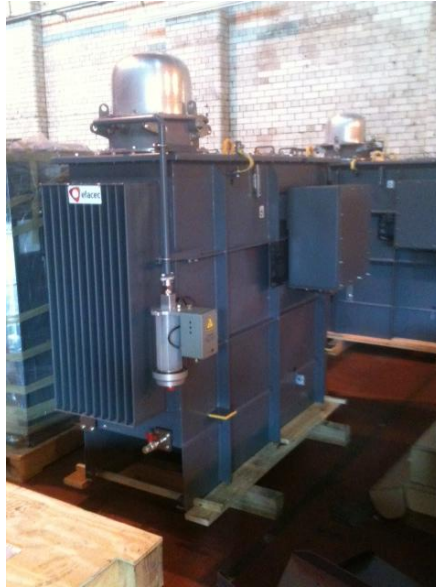
Figure 64: Transformer with OLTC installed for Landgate and Leicester Av substations
