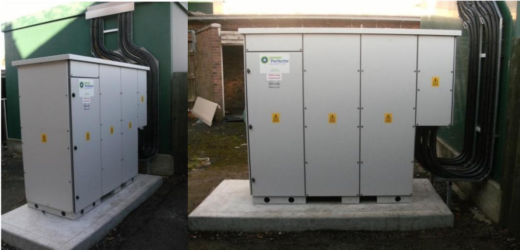
Figure 22: powerPerfactor unit installed at Edge Green Lane substation
