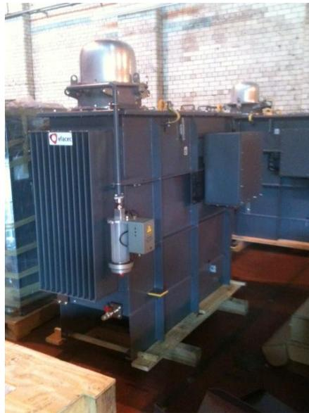
Figure 8: Distribution transformer with OLTC installed for Landgate and Leicester Av substations
