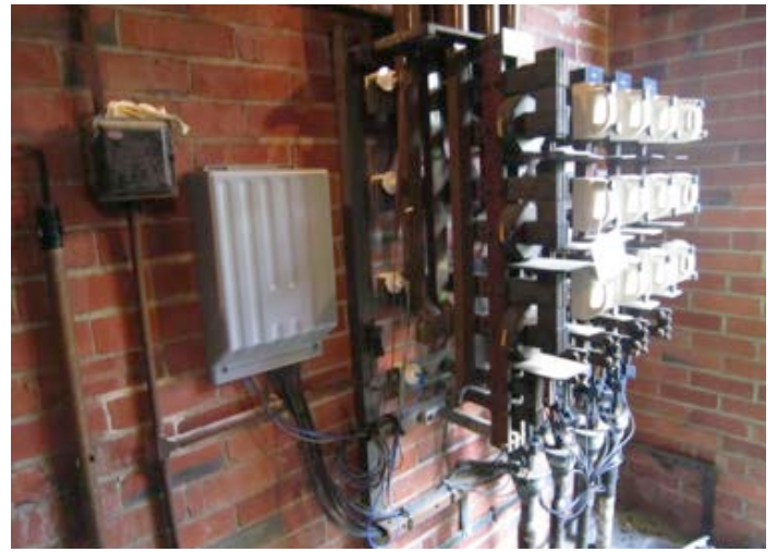
▲ Figure 18 – Substation Monitoring
