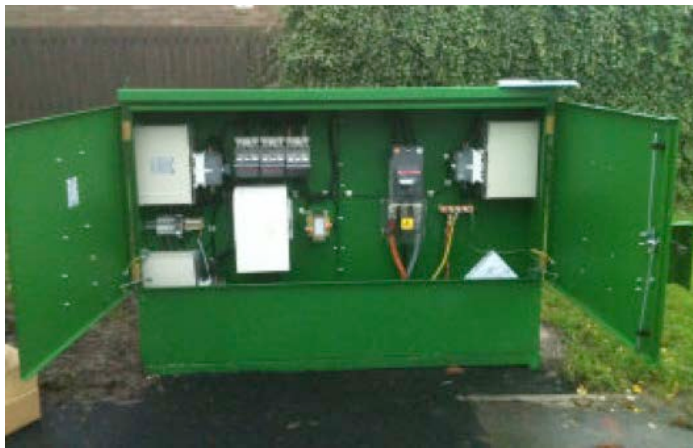
▲ Figure 8 – LV Capacitor
