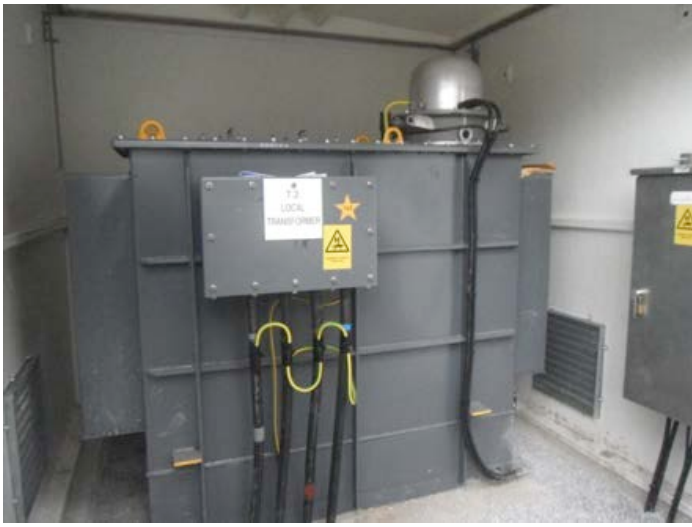
▲ Figure 1 – Distribution Transformer with on load tapchanger
