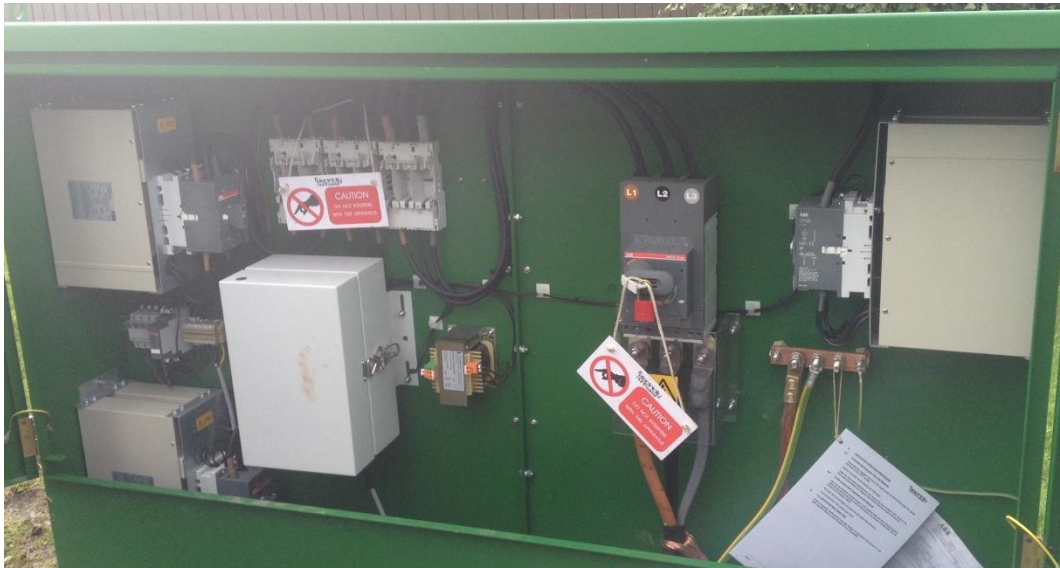
Figure 2 Capacitor bank in Leicester Avenue in feeder 69051565
