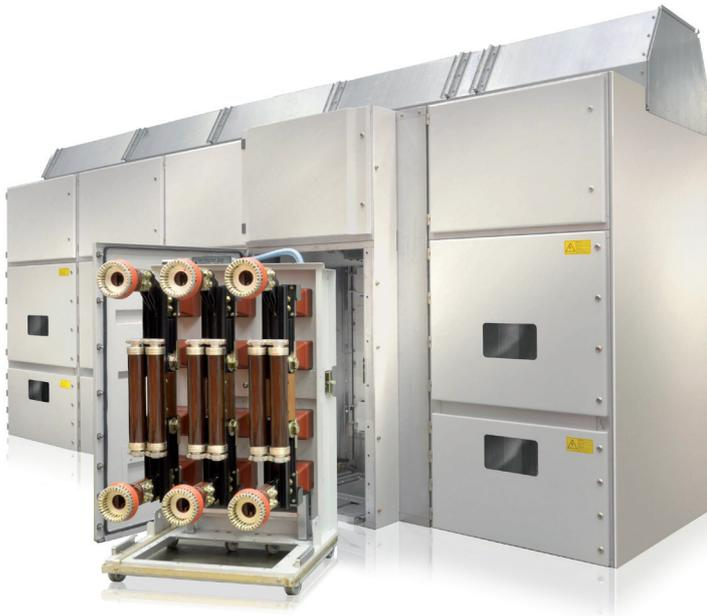
Truck mounted I<sub>s</sub>-limiter in a switchgear panel
