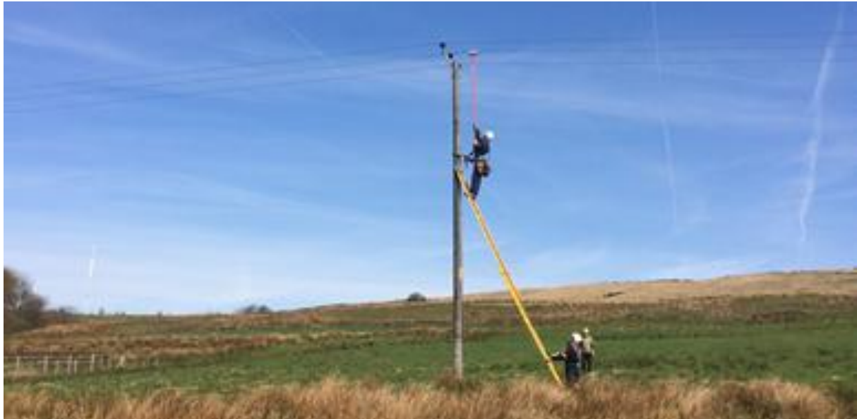
Figure 1.1: Electricity North West lines team installing a voltage measurement device using live line techniques
