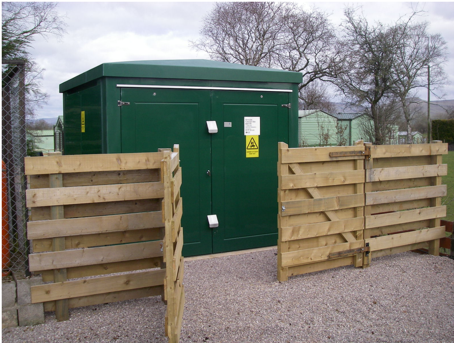
Substation (metal or plastic housing)
