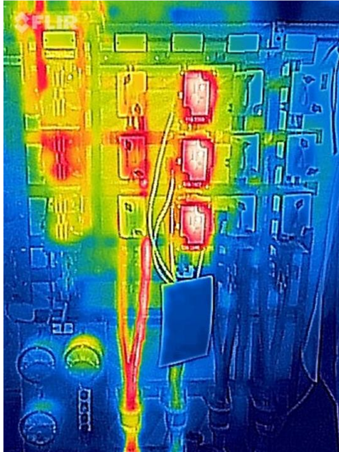
Figure 12: Thermal image of LV switchgear taken in Wentworth Road.
