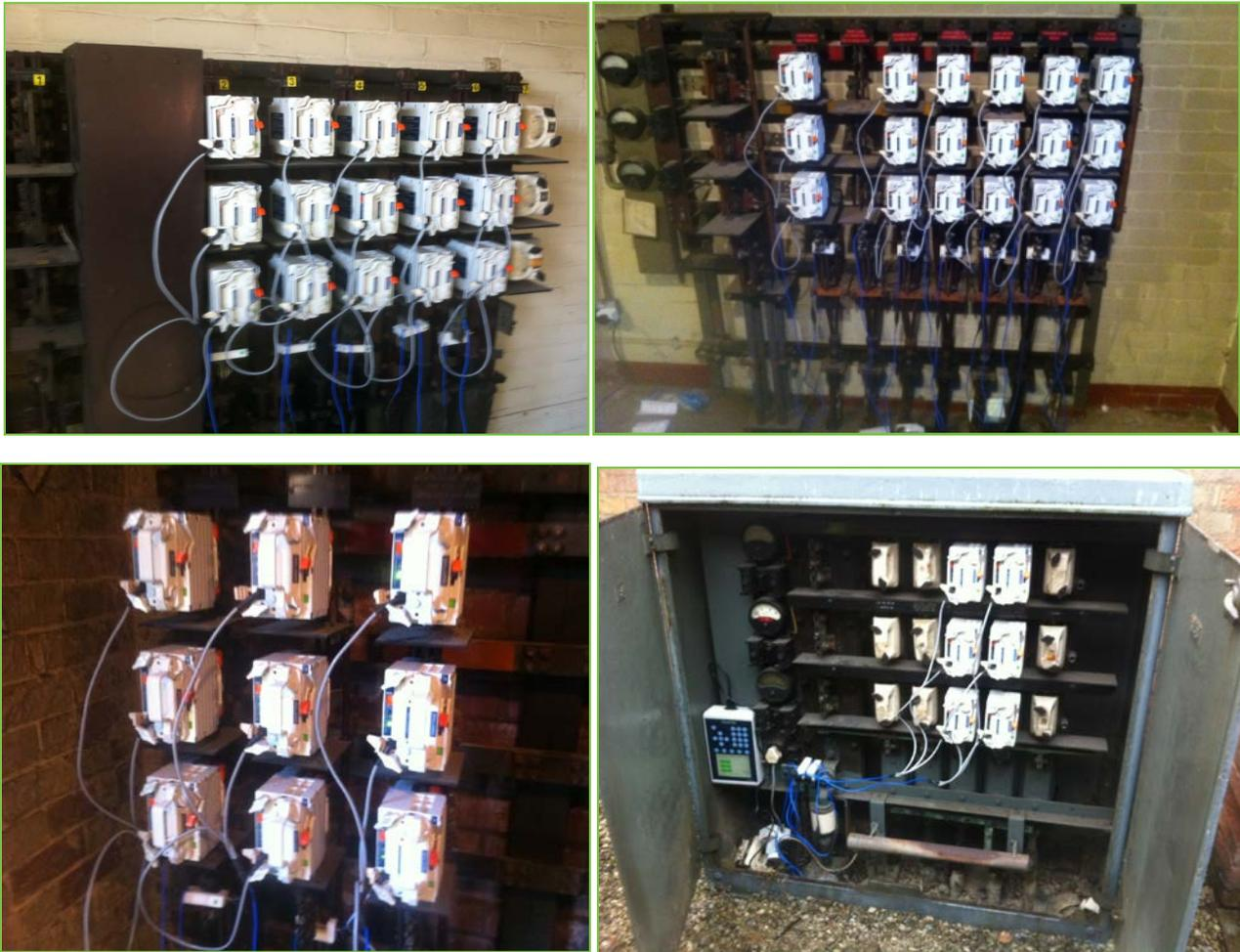
Figure 7-3 - Various Installation showing the types and variations of indoor and outdoor LV Feeder Pillars
