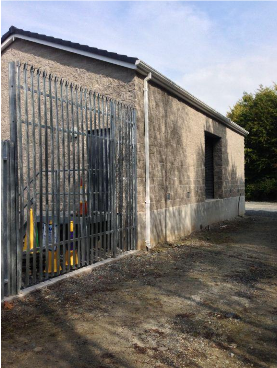
High voltage switch room under construction on a raised plinth. (Courtesy NIE)
