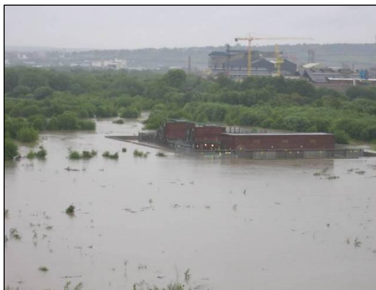
Photograph 1 - An electricity substation protected by flood barriers in the 2007 floods in the North East of England
