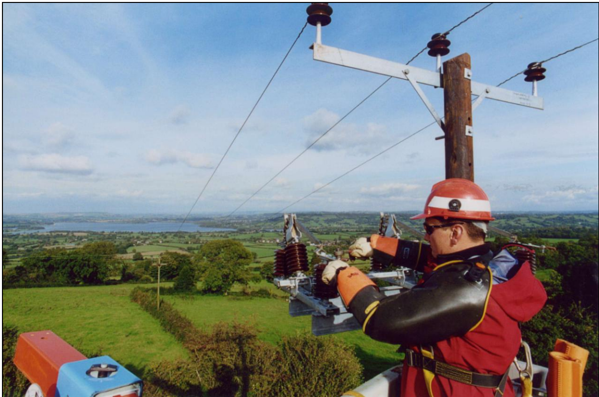
Photograph 13 – Hot glove live line working – personal protective clothing and equipment
