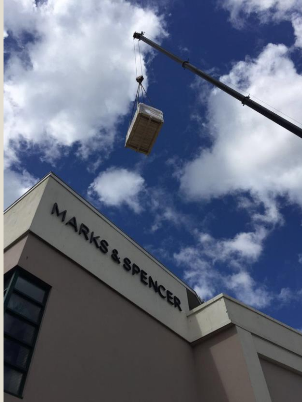
A shot taken by solar installers Joju
