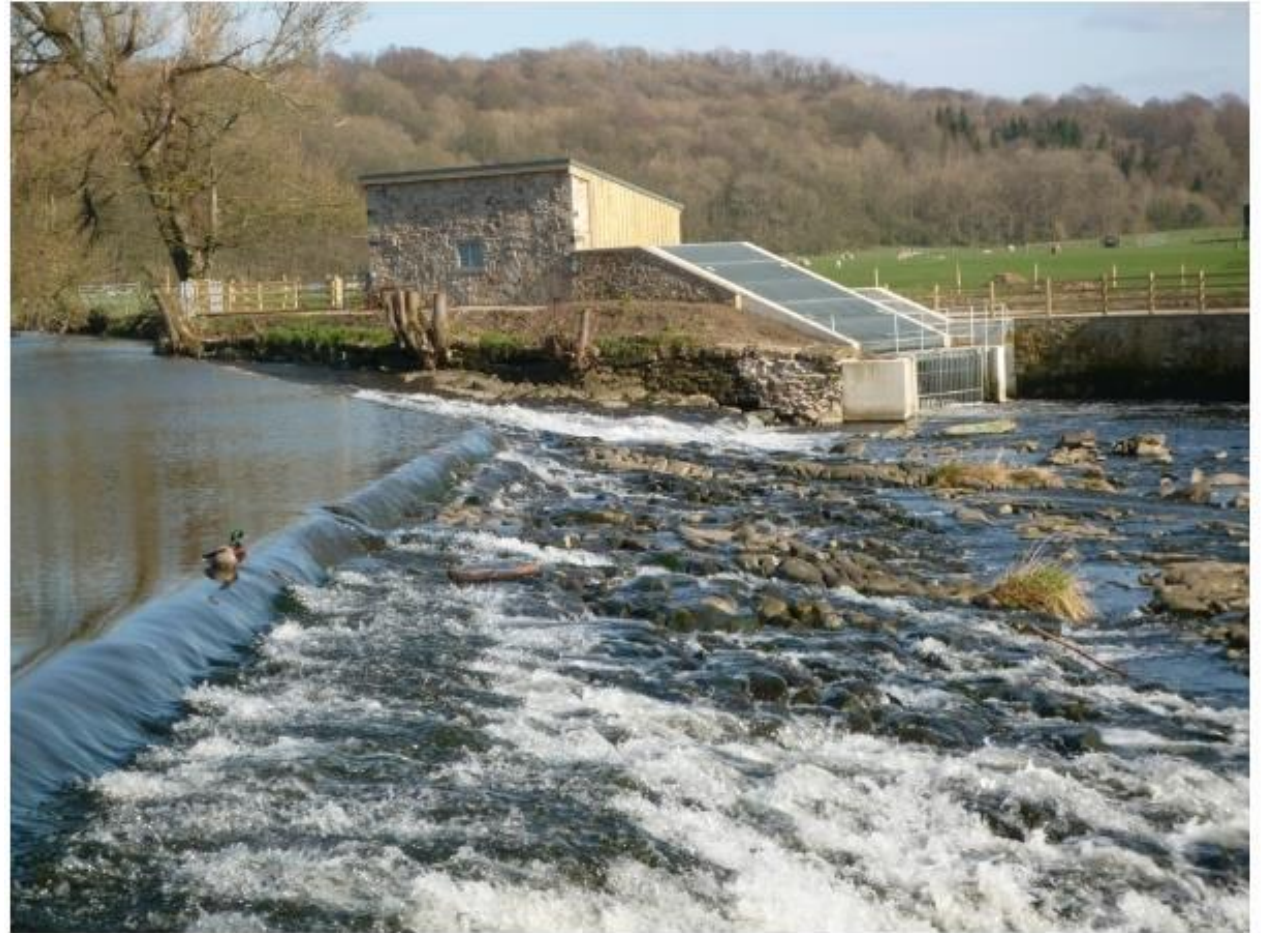
This 100kW hydroelectric generating plant on the side of the River Calder at Whalley, Lancashire began generating in November 2014.
