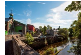
James Cropper Plc, Burnside Mills, Kendal, Cumbria Site of the 250kw Community Owned Solar PV project
