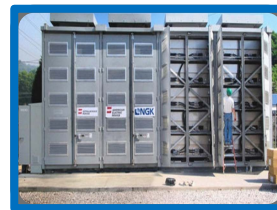
Network energy storage
