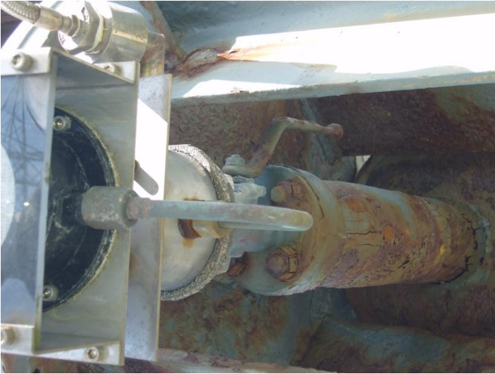
SF 6 Receiver showing corrosion at Peel
