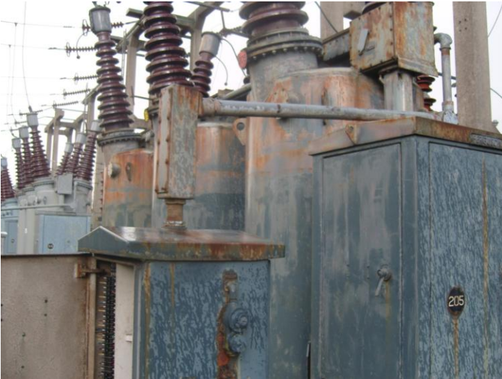
Corroded circuit breaker tank at Padiham
