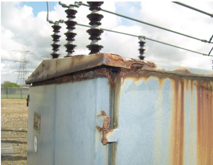
Heavily corroded marshalling kiosk at Peel
